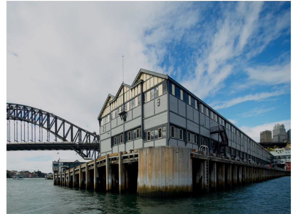
Top: Walsh Bay Piers 2 & 3 involved the RESTORATION and repair - above and below water - and conversion of 1912 - 1921 State Heritage Listed two storey, hardwood framed wharf and store-sheds to residential apartments.
